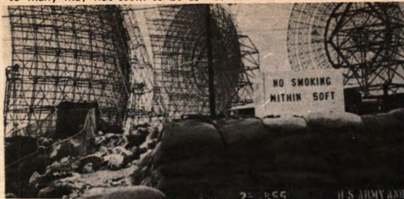
These 120-foot troposcatter antennas in Vietnam are similar to the ones being designed at Stanford.
